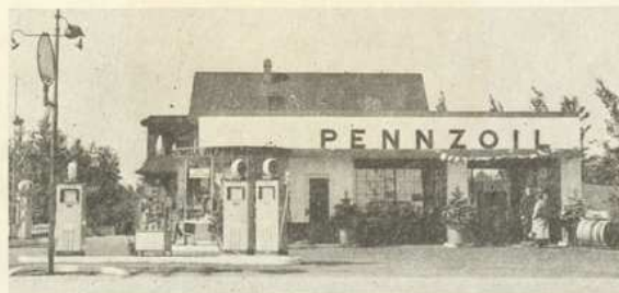
That's what Architectural Forum for February calls this station that faces General Electric's "university of light," Nela Park, East Cleveland, O. The station is owned by Columbia Refining Co., Cleveland, and is operated by Ed Bossman, a dealer.
